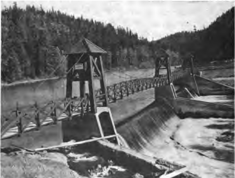
FIG. 96.—Sprague River Dam, Klamath Indian Reservation, Oregon.
